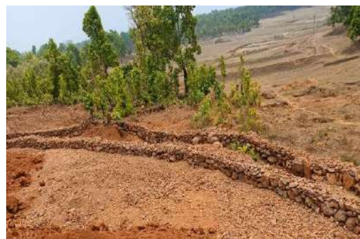
Photographs of garland drains and parapet walls
