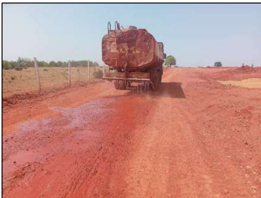
Water Sprinkling in haul road
