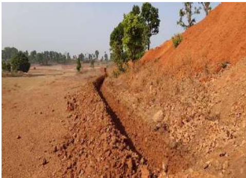
Photographs of garland drains and parapet walls
